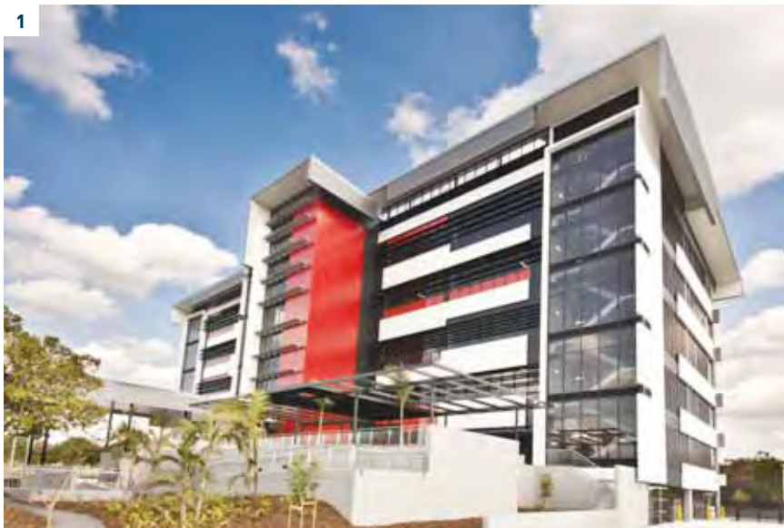
15 Lobelia Circle, opened in October 2012 and occupied by the Australian Federal Police, is the first office building in the International Terminal precinct.
